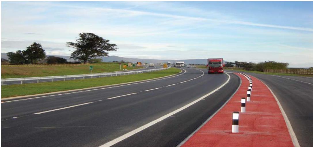
A66, Temple Sowerby, the finished bypass in use
